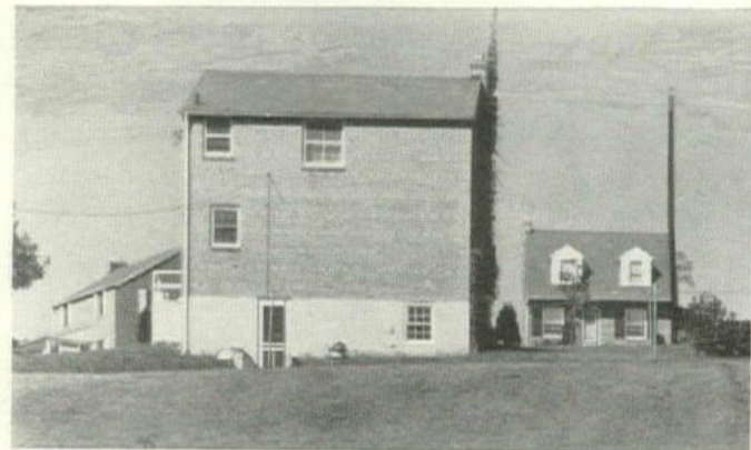
Before Hay designed for Seal & Turner, rear elevations on 1949 houses looked like this: tiny windows miss sweep of rolling countryside; poorly lighted basements are no invitation to indoor-outdoor living. Now see right.
